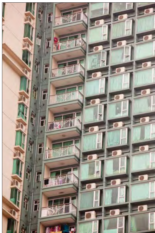
Air conditioning for urban buildings drives energy consumption upwards
